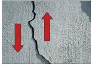
Uneven loading and settling of footing
